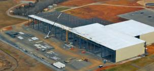
NBS can reduce or eliminate the need for independent crane columns. Many buildings can easily be designed to handle the loads imposed by the crane system. The elimination of the redundant crane structure often results in substantial savings for the building owner.
